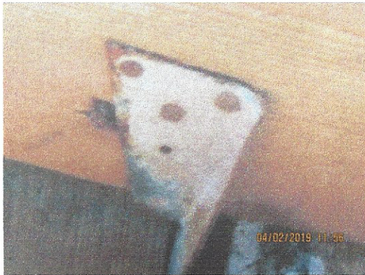
Hurricane clips visible with 3 nails RWA
