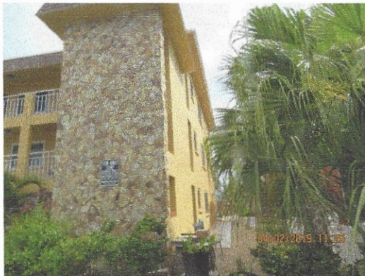
Right end of building
