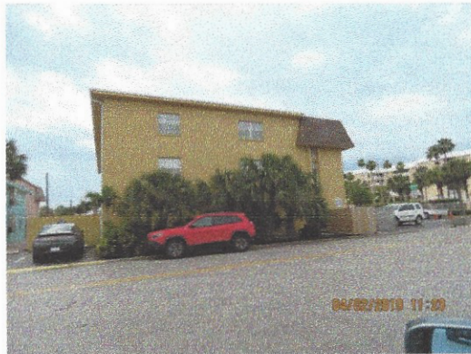
Left end of building
